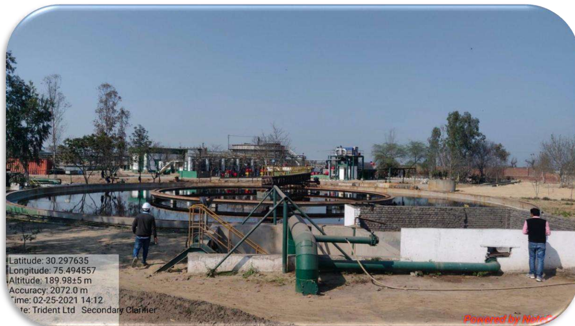
Fig 17 Secondary Clarifier
